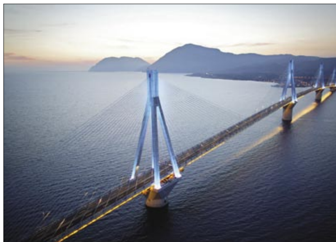
The cable-stayed Rio-Antirio bridge straddles the Gulf of Corinth connecting Western Greece and the Peloponnese
